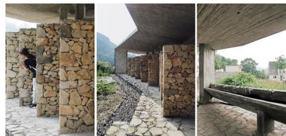
Figure 10: The bathhouse with a washing area facing the village farm (Photographed by Yao Li, Yang Xiaobo)
