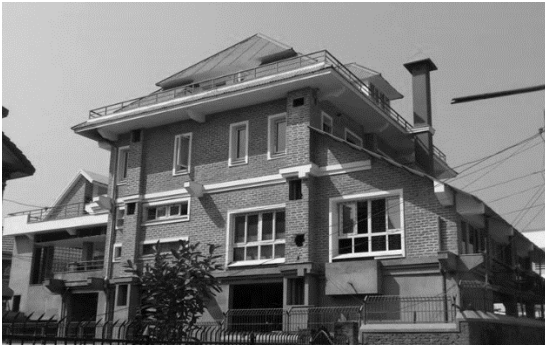
Figure 10: View of the modern green home
