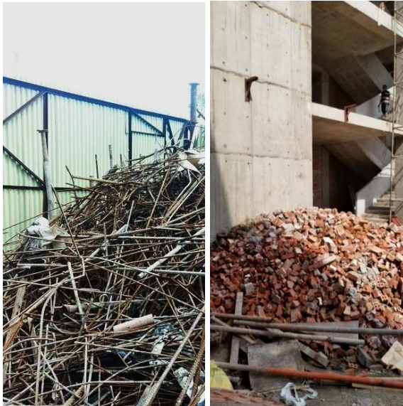
Figure 4: (right to left) rebar wastes at Blue Ocean Footwear Factory, Brick Bat leftovers at Golden Sky footwear factory. Source: Author
