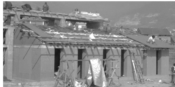
Figure 5: View of Mato Ghar during construction
